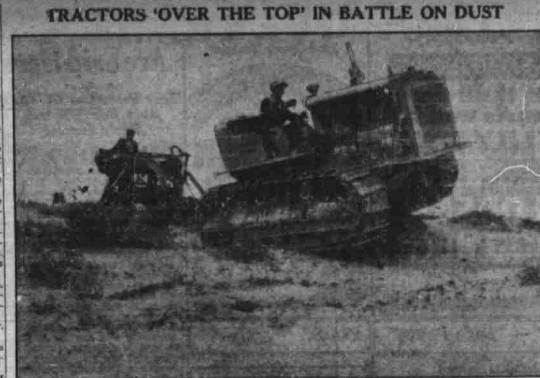
TRACTORS 'OVER THE TOP' IN BATTLE ON DUST It is determined warfare against a relentless foe—the tireless, soil-blowing winds—that farmers of the Southwest "dust bowl" and the government are waging. Here is one of the 50-ton tractors on the 26,000-acre soil conservation project near Dohart, Tex., trying to restore the land to tillable level by grading down sand dunes. (Associated Press Photo)
