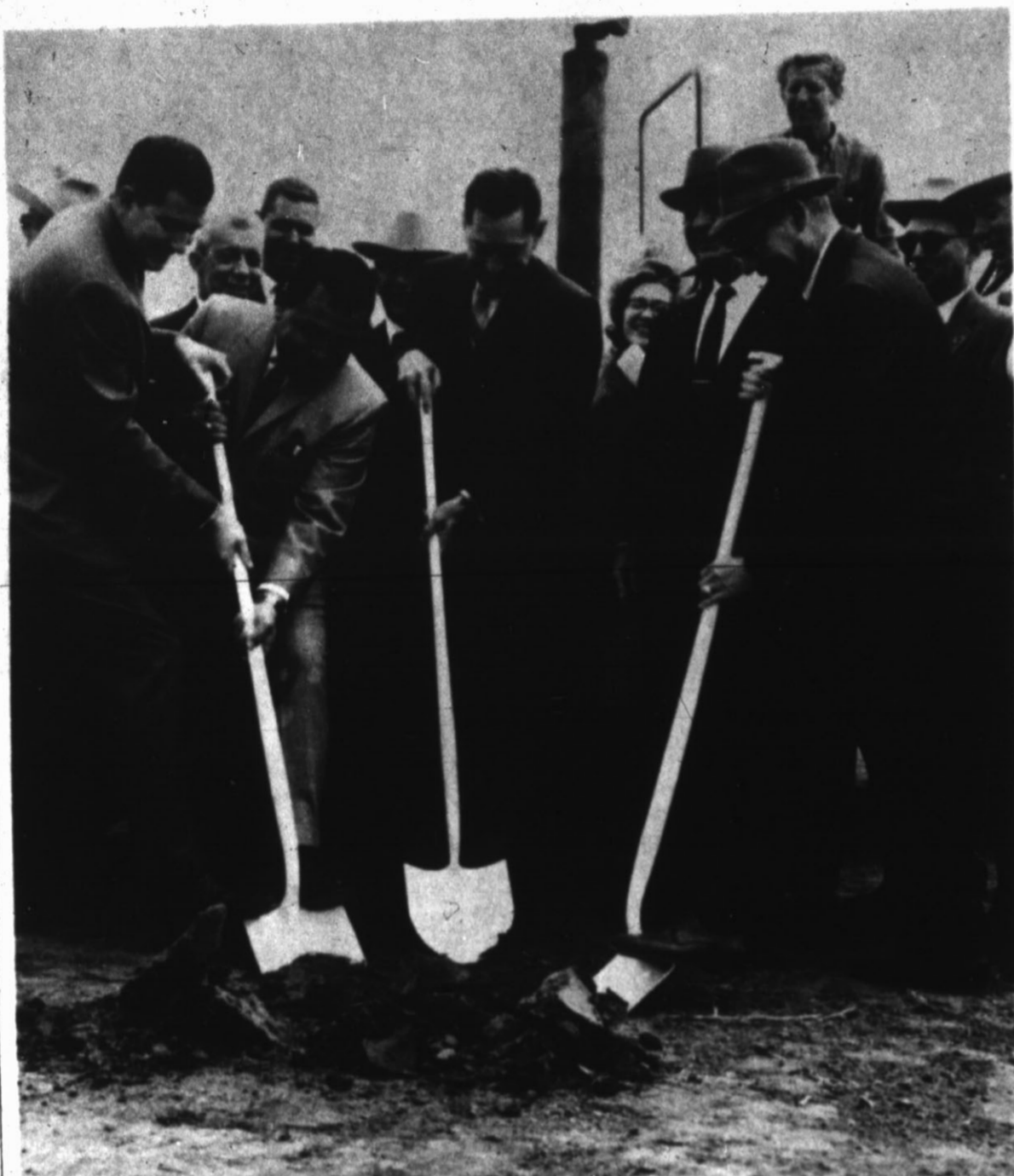
MALL OFFICIALLY UNDERWAY — With a phalanx of local and out-of-town dignitaries looking on, four men involved in the development of the Sugarland Mall Shopping Center here spade the dirt in a ground-breaking ceremony Wednesday morning. They are (left to right) Henry Huneke of Lubbock, president of the Mall corporation; Joe J. Aguilar of Lubbock, vice president; W. B. Rushing, developer; and James Walker, contractor. See story on page 1. (Staff Photo)
