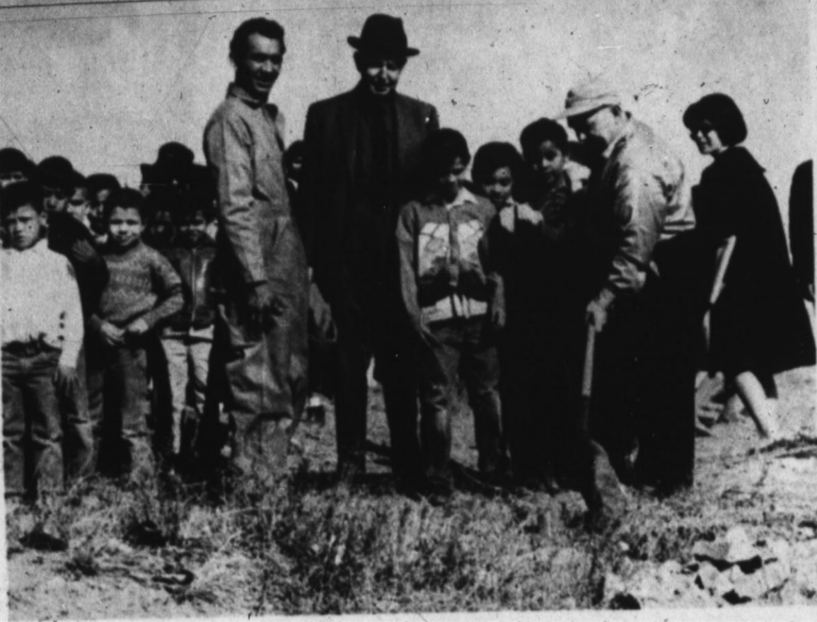
BREAK GROUND FOR PARK — Ground-breaking ceremonies were held this week at the Labor Camp on land donated for public use by D. W. Finlan. The lake area given will be used for a ball park and a playground, explained Bro. Chrys of St. Joseph's Mission. Shown here breaking the soil for a drainage route to the Tierra Blanca Creek are Armando Perez, Scoutmaster of Troop 145, D. W. Finlan, donor, and Bro Chrys. Looking on are boys and girls from St. Joseph's School. (Staff Photo)
