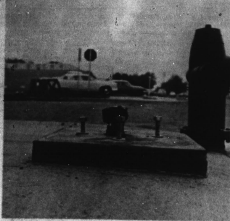
STREET LIGHTS? — Although one couldn't guess by looking at this picture, street lights are going up at Third and Miles. The covered outlet is for electricity. (Hereford Brand Photo)
