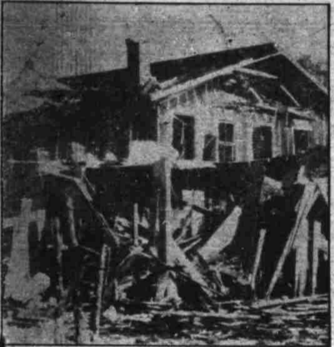
Fifty homes and buildings were destroyed or damaged, seven persons were injured and 75 were made homeless by a terrific explosion of 250 kegs of blasting powder and 20 kegs of dynamite stored in a building at Helenwood, Tenn. This photo is typical of the destruction caused. (Associated Press Photo)
