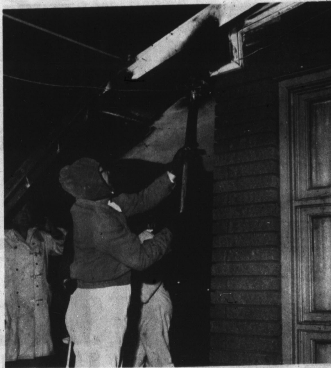
AN ELECTRICAL SHORT in the neon sign at the Lucky U Motel caused an early morning fire which is blamed for $3000 to $4000 worth of damage. The alarm, which sent volunteer firemen to the motel on West Highway 60, was turned in about 3 a.m.
