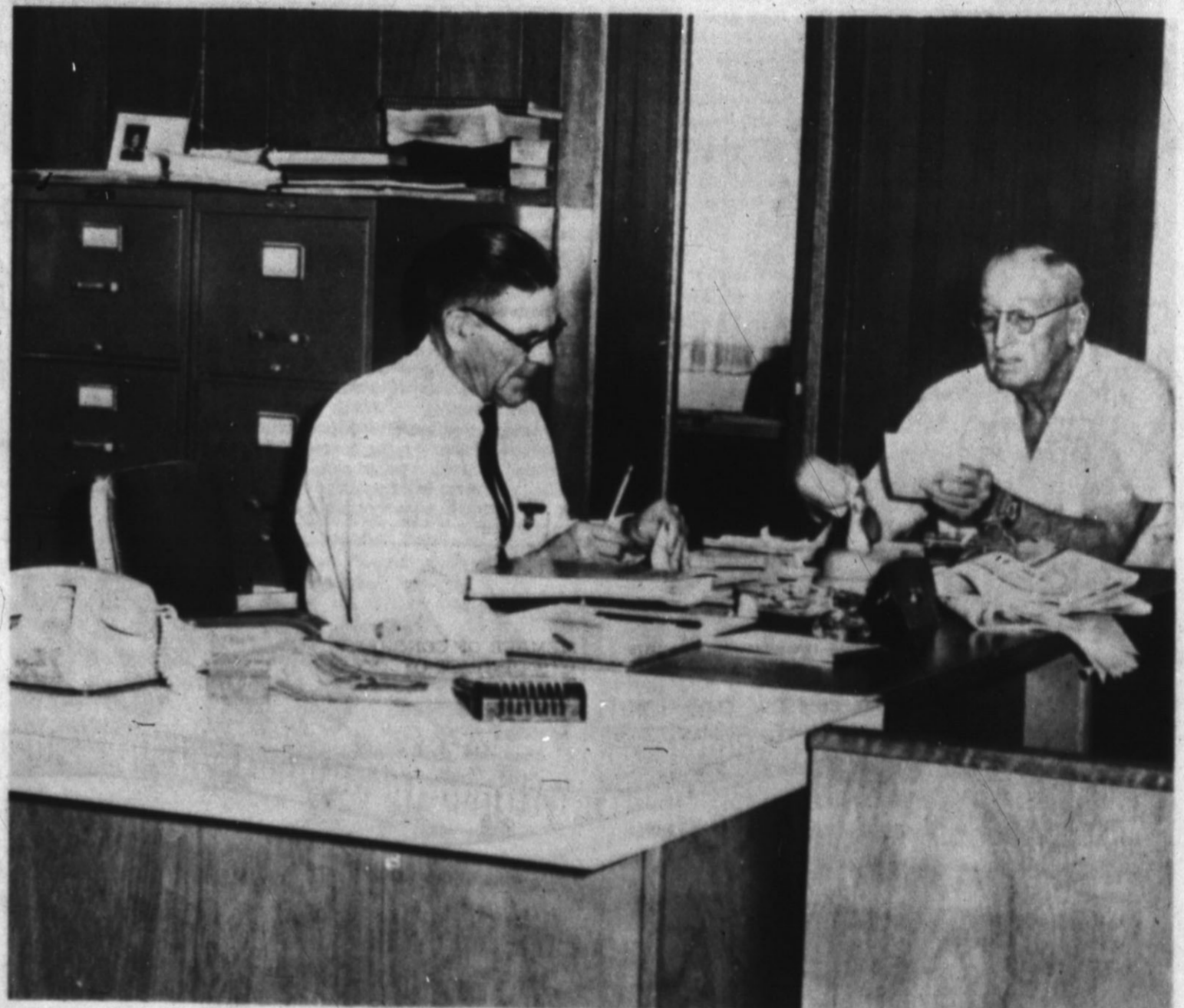
CONDUCTING BUSINESS — Wallace Shelton, left, and Jim Neill, newly appointed corporation court judge go over police business at the reception desk in the newly remodeled city hall. Shelton is a dispatcher for the Hereford Police Department.
