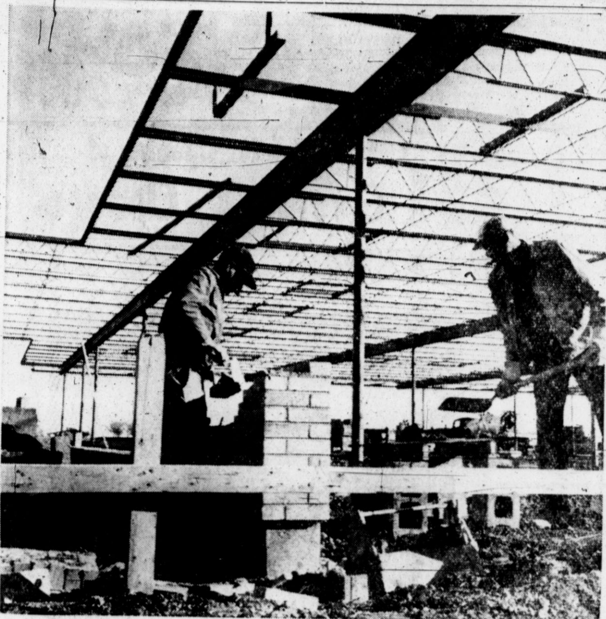
A STEEL LATTICEWORK covers a bricklayer and his helper as exterior walls start up on the northwest elementary school, presently under construction. The eight-room building is expected to be finished and ready for use next September and will provide facilities for the expanding residential area which is mushrooming with new homes. (Staff Photo)
