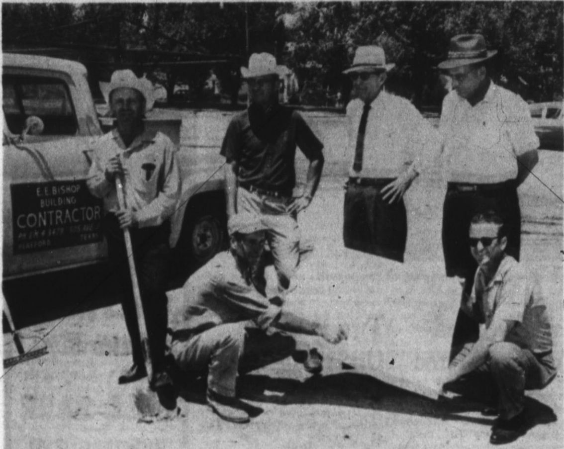
GROUND BREAKING — Ground was broken Monday at the corner of Jackson and Third for the new "Agri-Building" to house three U.S. government farm offices and a barber shop. Left to right are, standing, Sam Smith, owner of the building, Don Newman, SCS; Faust Collier, ASCS, and James Gouley, FHA. Holding the blueprints are E. E. Bishop, the contractor, and Troy Rowland, who will operate the Golden Spread Barber Shop. (Brand Staff Photo)
