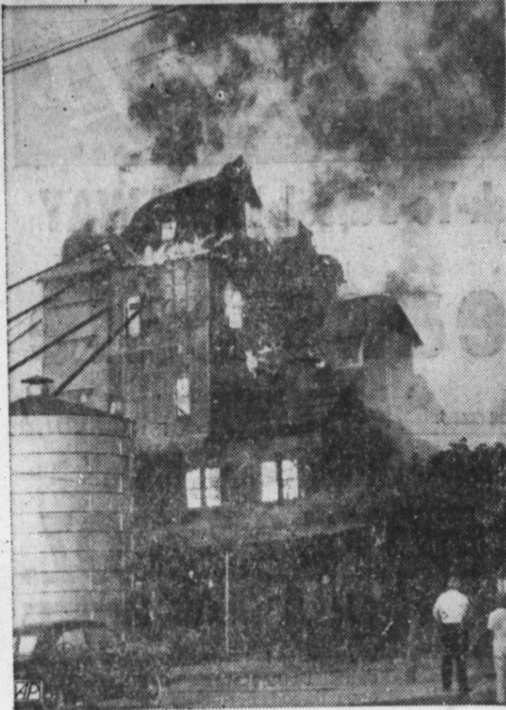
FIRE DESTROYS GRAIN ELEVATOR —Flames soar skyward during a fire which gutted the C. L. Green Milling Company grain elevator at Winters. Damage was estimated at $100,000 and about 12,000 bushels of oats were also destroyed. The fire is believed to have started by a dust explosion in the top and quickly engulfed the building. The fire came at the start of the first good grain season in this section of West Texas in seven years. (AP Photo)
