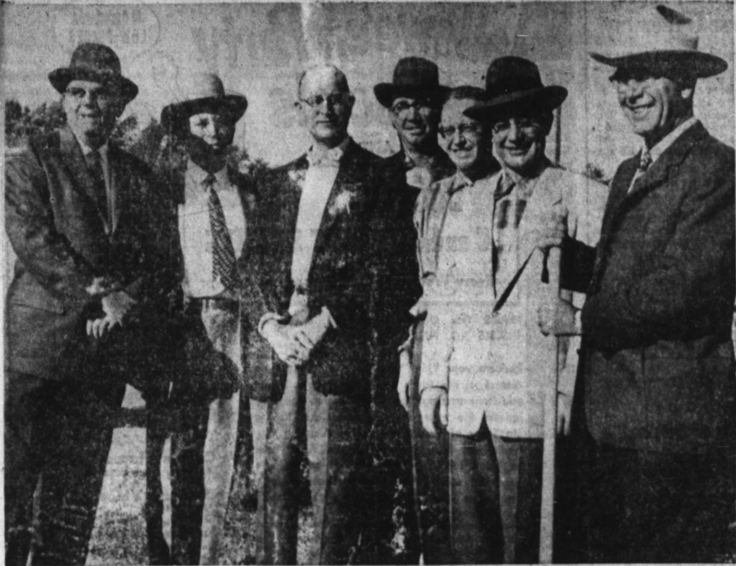
START "EMERSON 4 BUILDING"—Mayor Henry Sears, right, turned the first spadeful of dirt at the ground breaking ceremonies of the new Southwestern Bell Telephone Co. building on Miles St. When completed late in 1957, the "Emerson 4 Building" will house equipment to give the area the most modern telephone service. At the ceremonies were Townsend Douglas, left, Chamber of Commerce president; A. O. Thomas, Southwestern Bell's district manager; R. R. Wills, Troy Moore, Neil Cooper and Raylan Evans, city commissioners. (Staff Photo)
