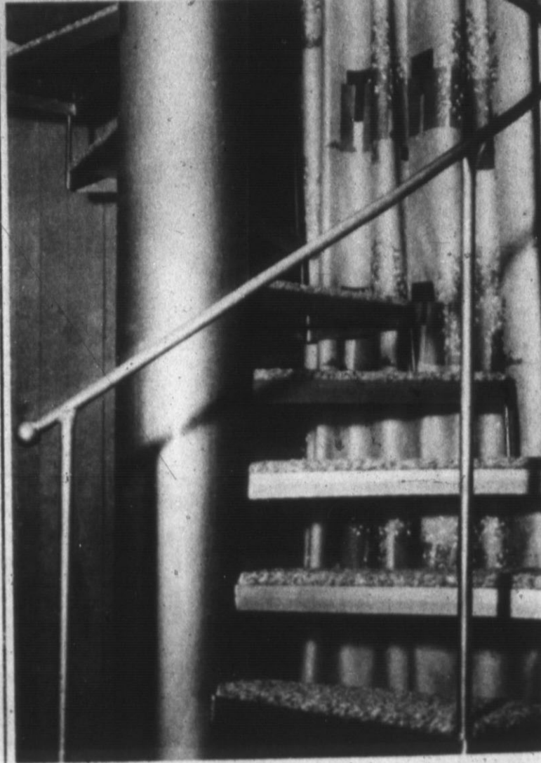
where there are two bedrooms and a bath. A window extending from the lower to the upper level forms a background for each stairway. On the upper floor the center post supporting the stairs terminates in a place for a potted plant at the end of an openwork iron balcony.
