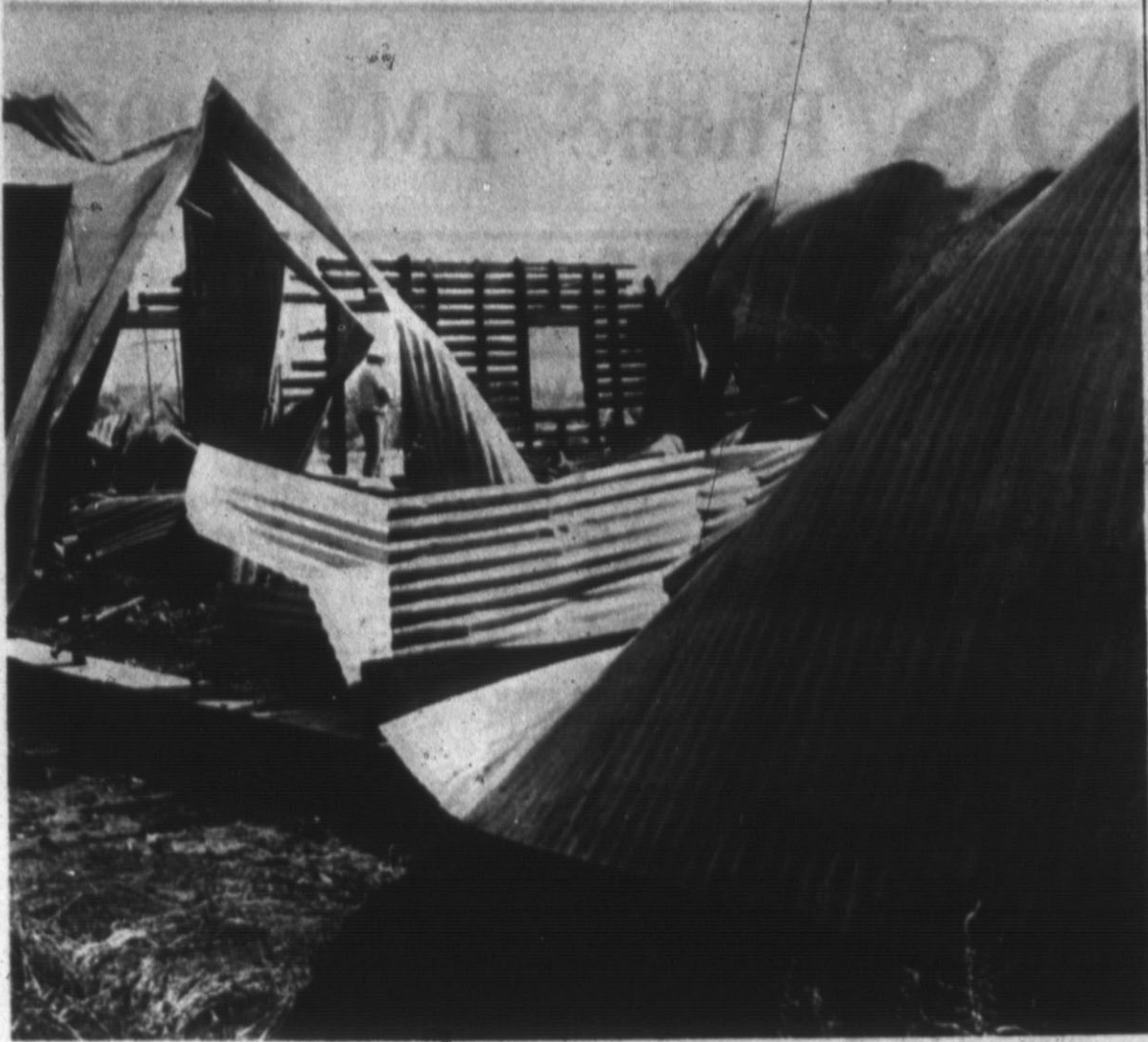
SALE BARN BURNS — A huge metal and wood sales barn on Austin road southeast of Hereford, was virtually destroyed by fire at 2:10 Friday morning. Fire Marshall Clay Angelo estimated the loss at $15,000. Firemen had to pump water from a creek a quarter-mile away. The building was leased to Norman Frank who conducted Thursday sales. A small restaurant, owned by Wayne Jenness, also was destroyed. (Brand Staff Photo)
