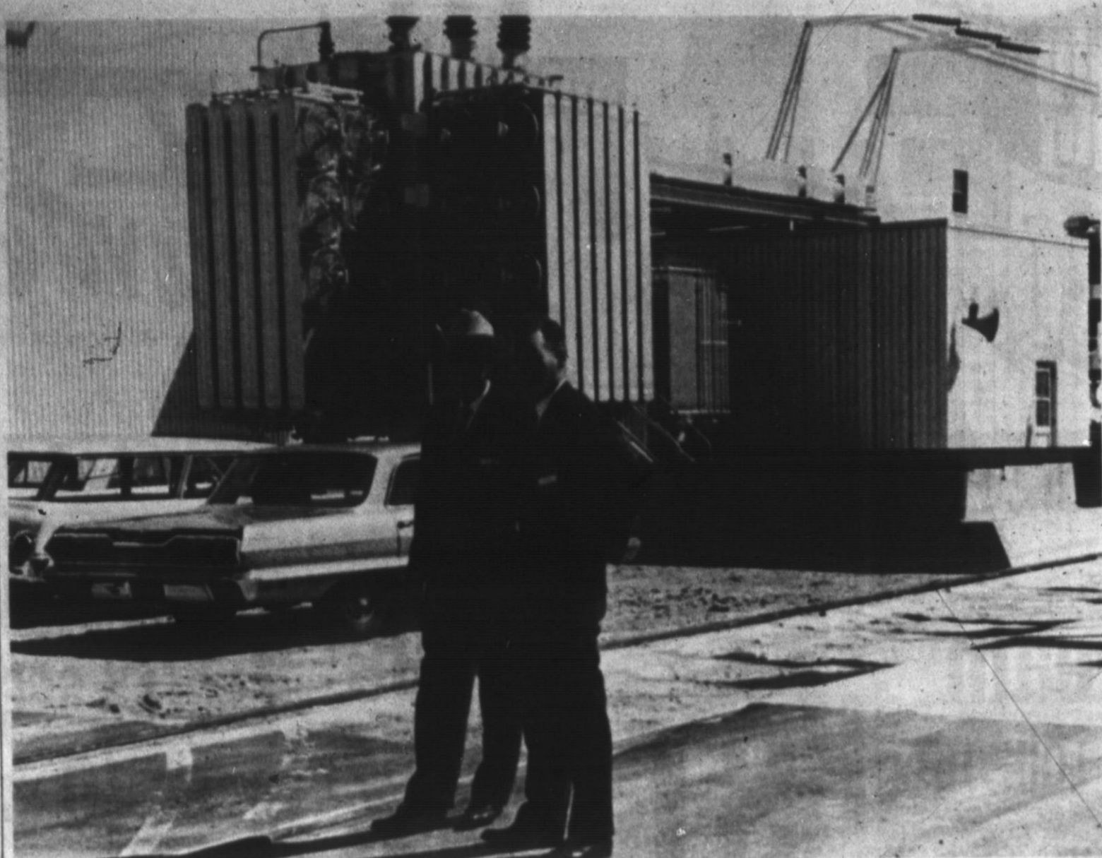
ATTEND OPEN HOUSE — Albert Maxwell, left and Jerry Detwiler of Hereford look over the $43 million dollar Plant X located at Earth. Business leaders from throughout the area were guest Friday of Southwestern Public Service Co. at a barbecue and open house at the gigantic West Texas generating plant. (Brand Staff Photo)
