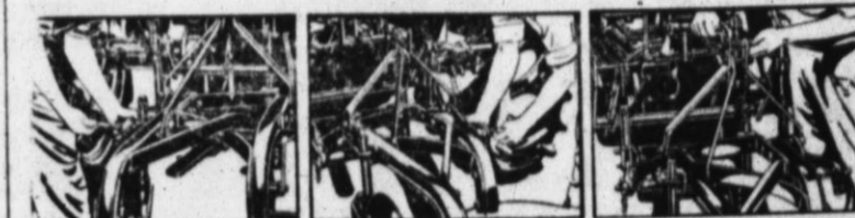
Snap on the left-hand draw The right-hand draw strap . . . and the adjustable upper link strap . . .
