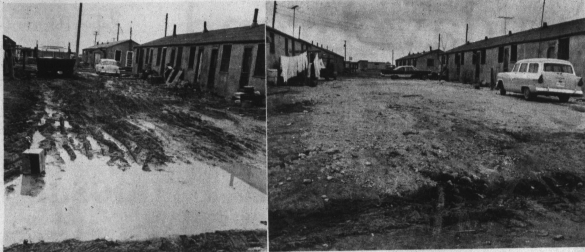
BEFORE AND AFTER are dramatically illustrated in these two photos from the Labor Camp. Picture at left shows problems residents face with mud and drainage. At right, conditions are improved by grading ditches and putting caliche in around the barracks. This is just part of an independent project to improve general conditions at the camp.
