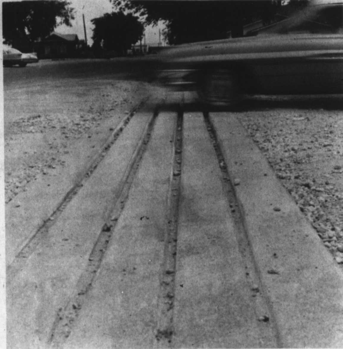
THE FIRST OF ITS TYPE, this ribbed or corrugated valley has been installed at the intersection of Fourth St. and Witherspoon. It has been placed at the intersection by the city in an effort to disperse traffic more smoothly and control excess water. (Staff Photo)
