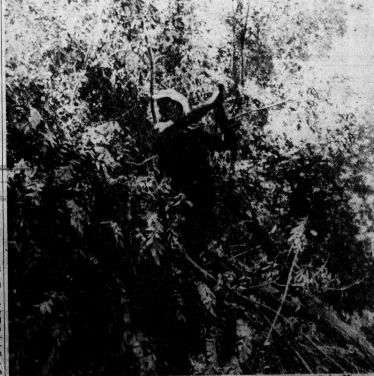
A FOREST OF TREES, 21 in all, was being removed from the Deaf Smith County Courthouse square this week in order that the grounds could be landscaped with grass shrubs and ornamental trees. Jack Messer had charge of the operation, using bulldozers and winch trucks to pull the 50-year-old elms. Workers armed with saws and axes then cut the giants into small pieces for removal. (Staff Photo)
