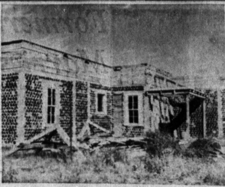
QUART OIL CANS was used to build the residence-greenhouse of Mr. and Mrs. J. R. Daniel at 213 Higgins St. The house was built during World War II when lumber was not available for constructing houses. Cement plaster holds the cans together and the outer wall is stuccoed. (Staff Photo)
