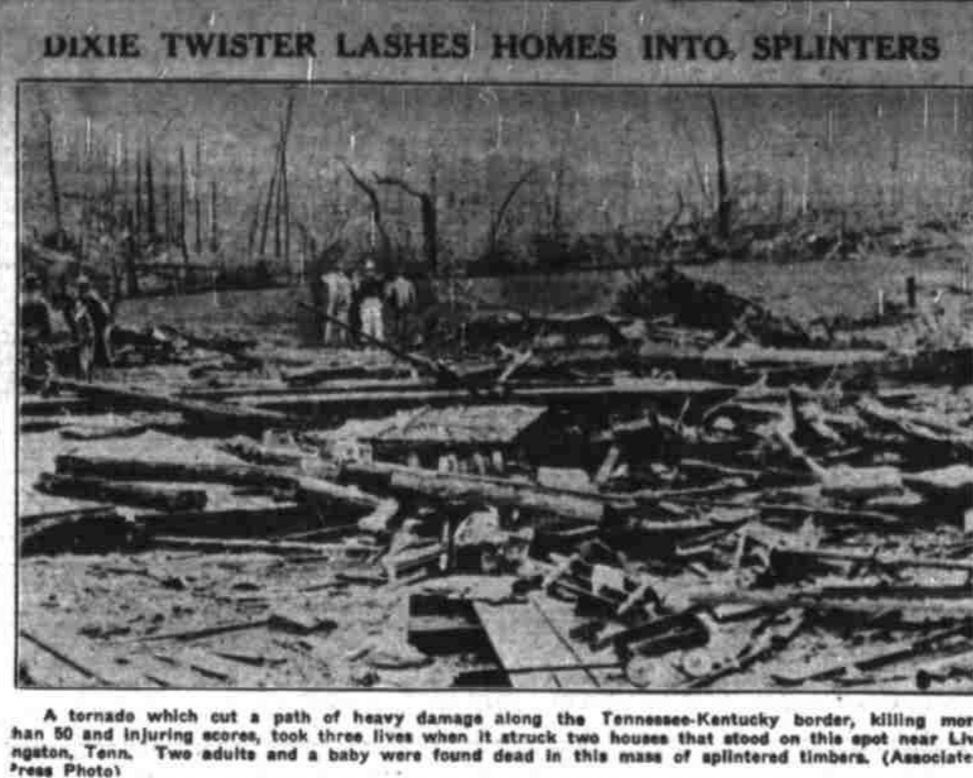
A tornado which cut a path of heavy damage along the Tennessee-Kentucky border, killing more than 50 and injuring scores, took three lives when it struck two houses that stood on this spot near Livingston, Tenn. Two adults and a baby were found dead in this mass of splintered timbers. (Associated Press Photo)
