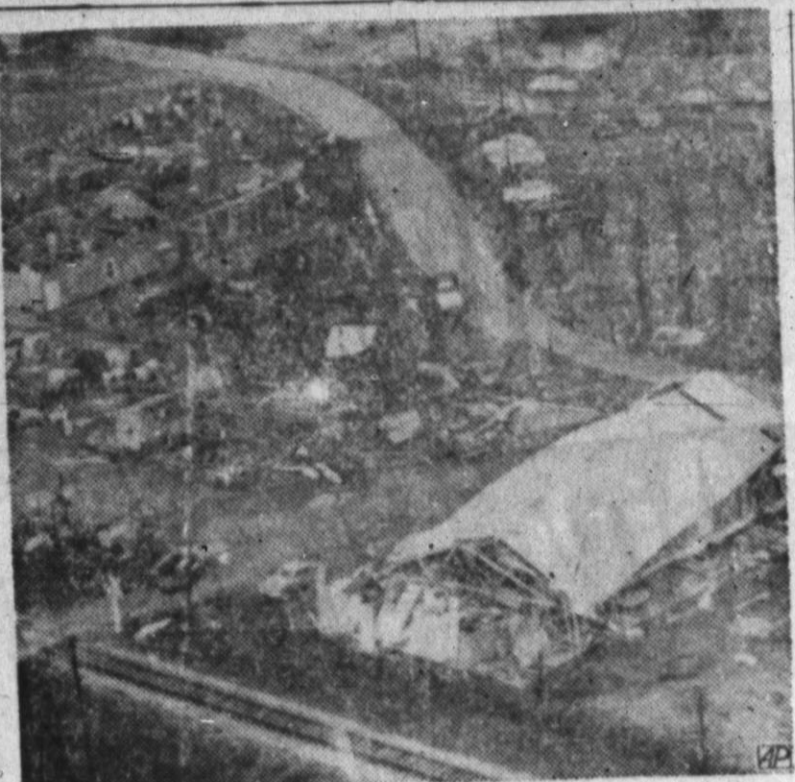
TORNADO DAMAGE—The broken shells of two buildings and the rubble of another bear mute testimony to the violence of a tornado that ripped through Bryan causing heavy property damage. The twister damaged over 200 homes and narrowly missed Texas A&M College and the Bryan Air Base. (AP Wirephoto)
