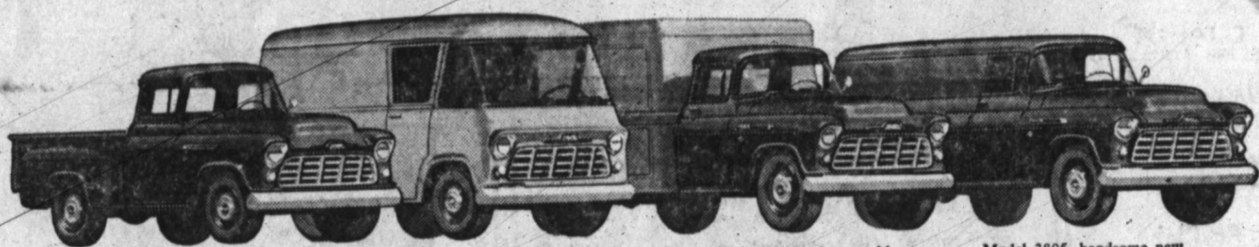
New 3000 Series truck, Model 3104, a 1/2-ton pickup. New 3 1/2-ton Forward Control chassis, Model 3442. Model 3803, 1-ton, shown with refrigerator body. Model 3805, handsome new 1-ton panel.
