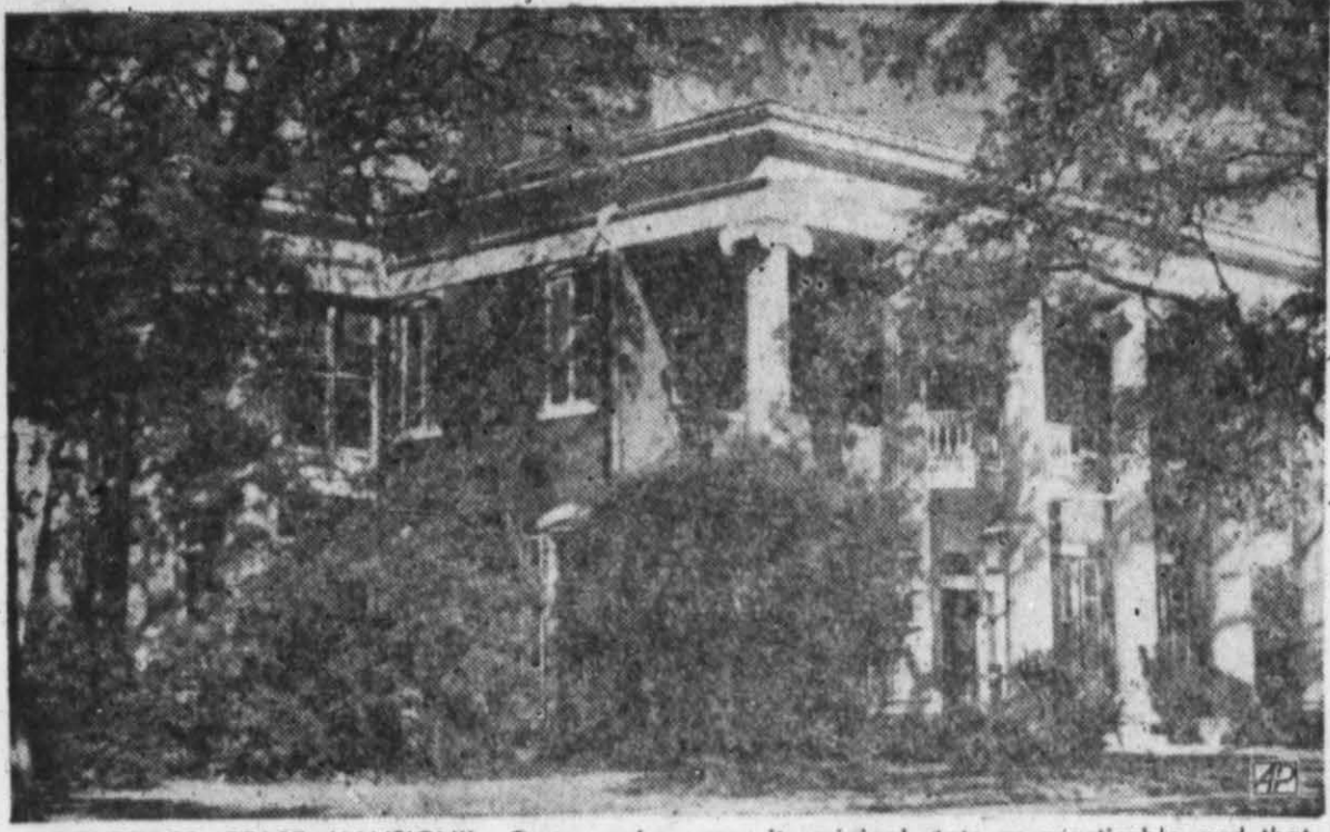
"GOVERNOR PEASE MANSION"—Gov. and Mrs. Allan Shivers announced in Austin they had purchased the 103-year-old historic house there known as the Governor Pease Mansion. Shivers said some remodeling would be needed but the house would be preserved in as
