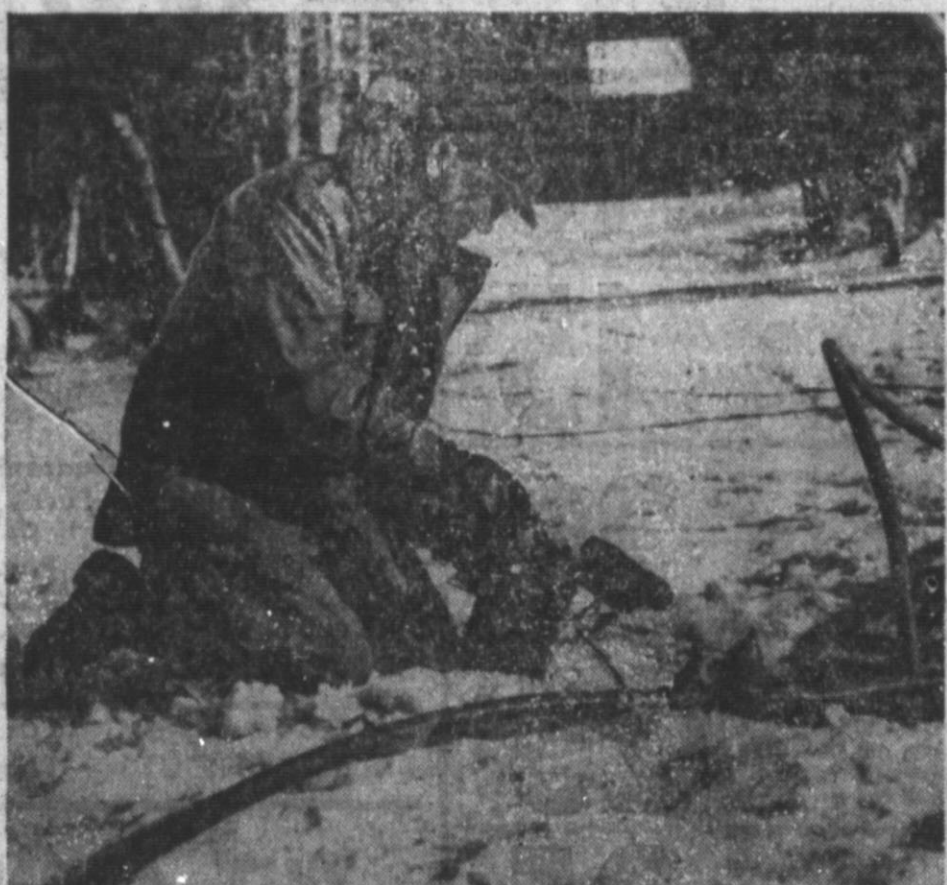
It's bitter cold morning, and Frank Eck, builder of snow-making apparatus, keeps machine in operation by warming up valve with kerosene flame.
