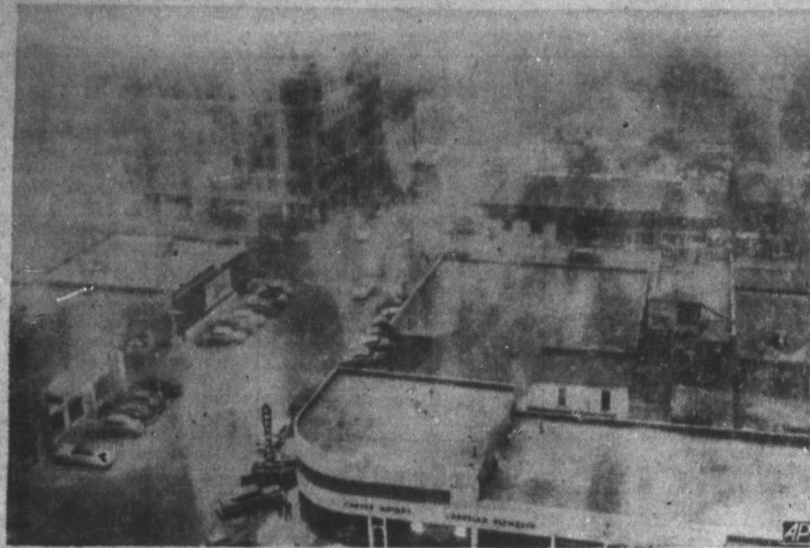
A SPRING DAY IN AMARILLO -- A dust storm whipped across Amarillo, and brought visibility to around a city block. This particular scene, taken from the top of the Her- ring Hotel looking South to the Capitol Hotel, when dust turned into rain and then snow. (AP Wirephoto)
