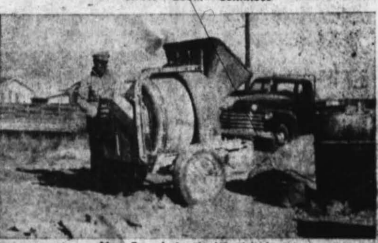
New Foundation in Westhaven
