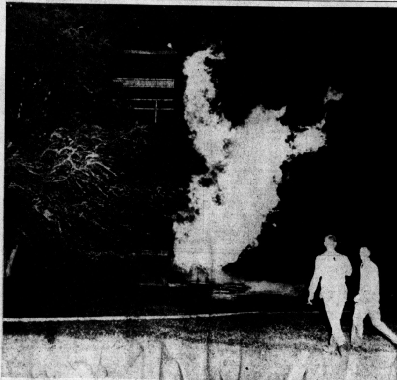
LOOKING LIKE A RUNAWAY GAS WELL, the Bovina school building gushed flames Thursday night during the fire which completely destroyed the combination grade and high school which had been used since the beginning of school by some 325 students, a higher enrollment than that which the school
