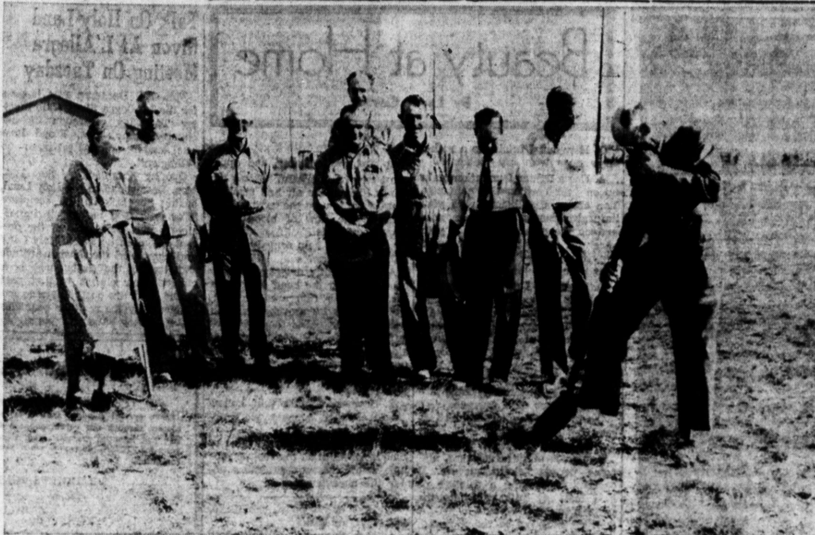
THE GROUND BREAKING of the new Wesley Methodist church, which will be located on Irving street, was held Monday morning. The laying off of the church began Monday. The expected completion date is December 15. Only one of three parts of a master plan will be built now. It will be the
