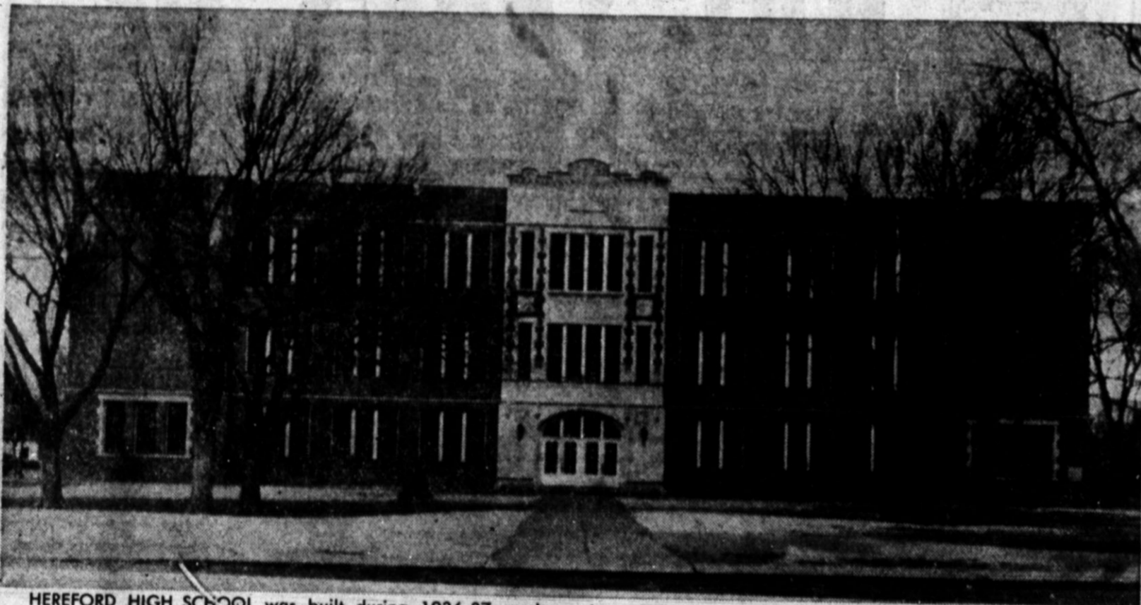
HEREFORD HIGH SCHOOL was built during 1926-27, and has had occasional modernizing work done on it through the years. When the new High School is completed, this school will be used for Junior High. Rewiring of the school, which was begun before Christmas, was scheduled to be completed Saturday. Superintendent George Graham says
