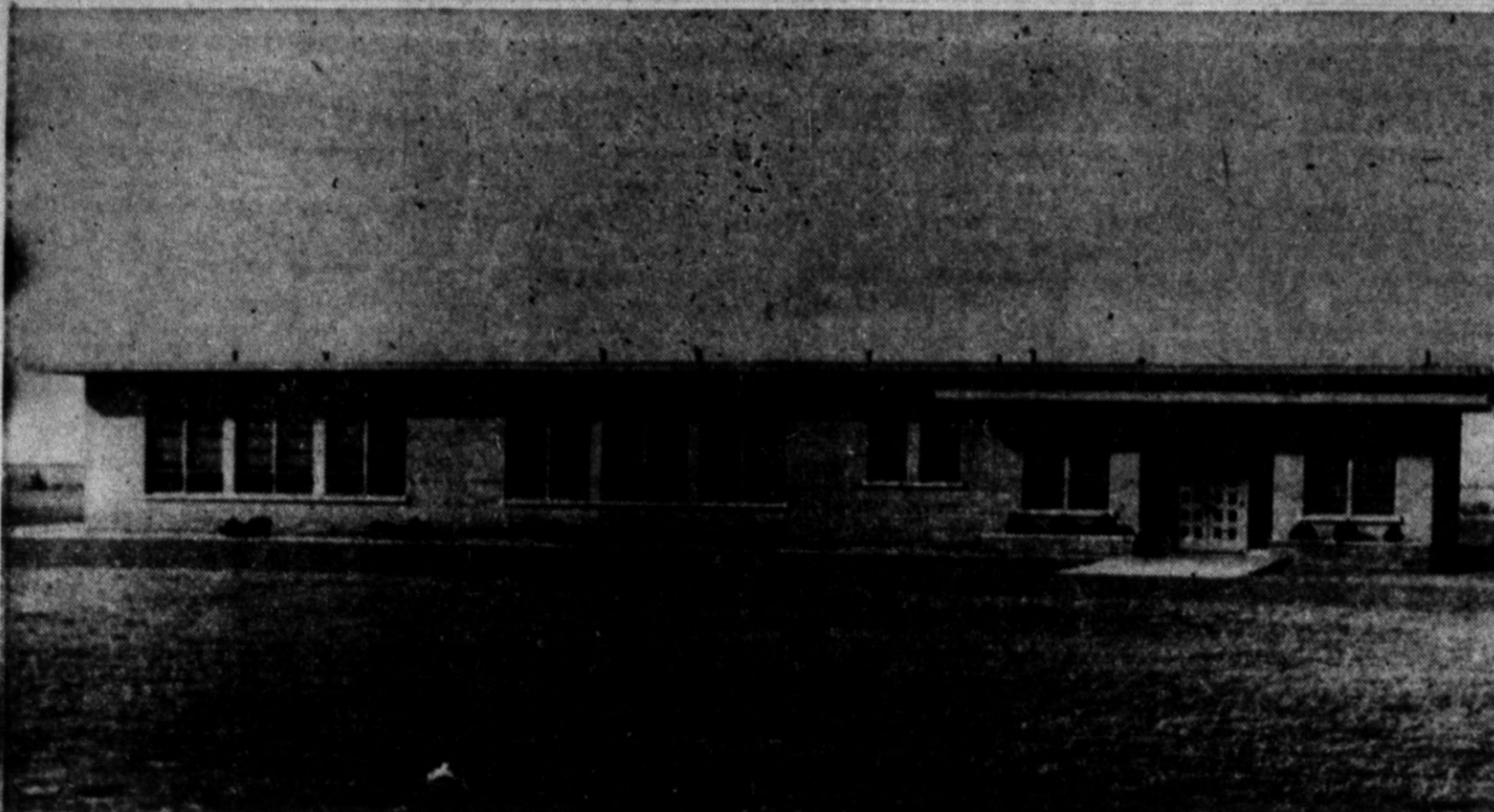
WALCOTT SCHOOL, which serves the Walcott Common School district in the western part of the county, is some 24 miles west and 7 1/2 miles north of Hereford. Classes have been held in the new building for the last three years. E. F. Baker is principal, and Mrs. Kyle Oliver Baker and Miss Lillian Fisher are teachers. There are 55 students
