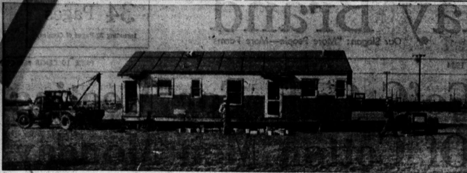
IT ISN'T VERY PRETTY right now, but the Hereford Rider's Club has plans which will make this building so different it will hardly be recognizable when the work is finished. The building was set down near the Rider's Club arena, and remodeling work is to begin immediately. (Staff Photo)
