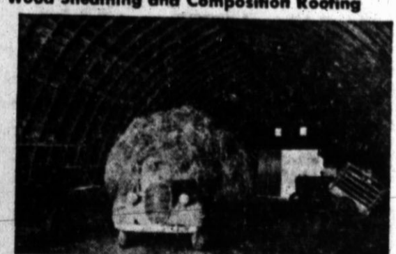
Every post-free interior offers great flexibility in a variety of uses. Rilco Rafters building may be used as a machine shed --with temporary partitions it will serve as storage structure or loading dock.
