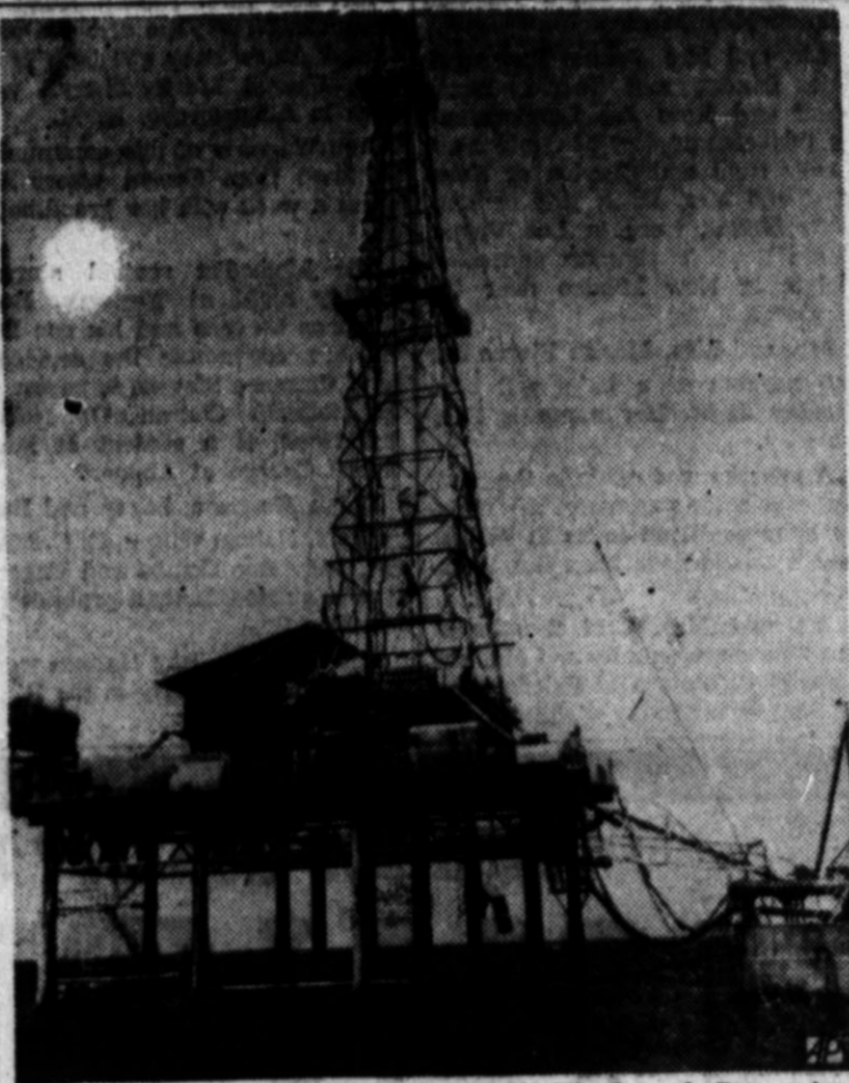
TIDELANDS PRODUCER - Standard Oil Co. of Texas has brought in the first producing tidelands well since the state's title to the offshore lands was upheld. The well is 1 1/2 miles off Padre Island in Kleberg County. It had an official 24-hour flow of 348 barrels of clean 39.5-gravity oil. The flow was through 12/64-inch choke from upper Frio perforations at 7,760-66 feet in 7-inch casing at 9,500 feet, with a total depth of 8,980 feet. (AP Photo).
