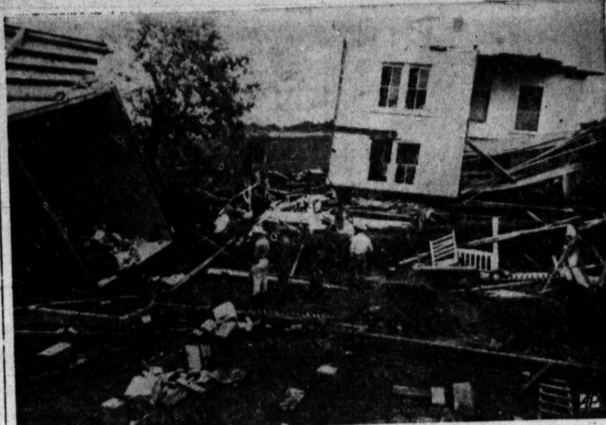
DEMOLISHED IN STORM'S PATH - Six persons were in the Otto Koerth home at La Bahia, 15 miles west of Brenham, Texas, when a tornado picked up the house, tore it in half, and threw one of the pieces end-over-end. The doors were blocked or high in the air, forcing the occupants to escape by windows. Miraculously, no one was hurt seriously, but livestock were killed in the yard. The storm damaged nearby houses and barns to a lesser extent. (AP Wirephoto)
