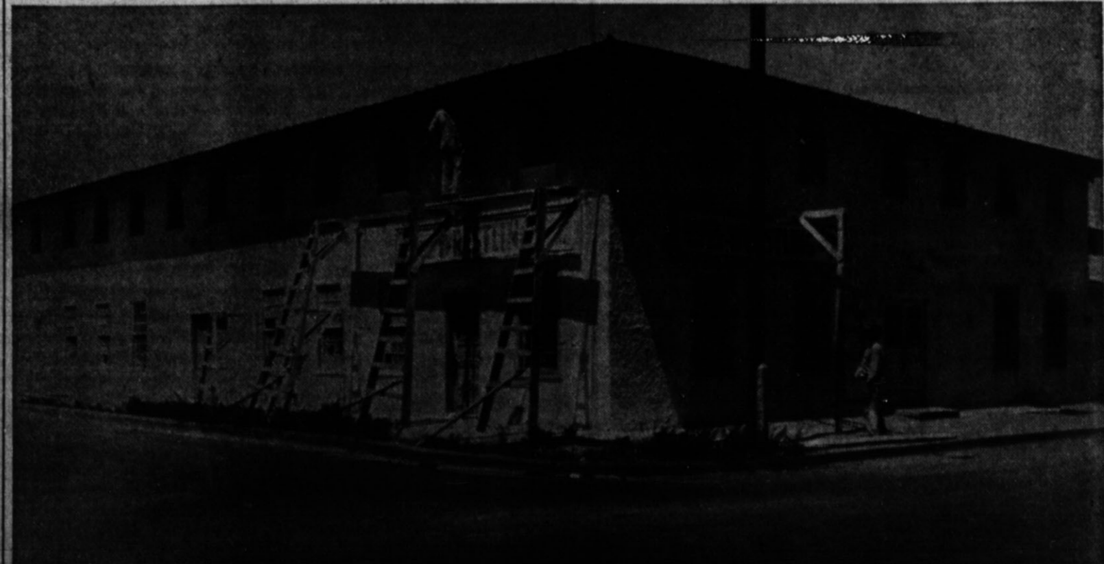
STUCCOING OF THE WEATHER-BEATEN exterior of the Bull Barn progressed rapidly during the first part of this week, changing the color from dirty cream to a gleaming white. Bob Gilbert, working on the scaffold, said that the building will
