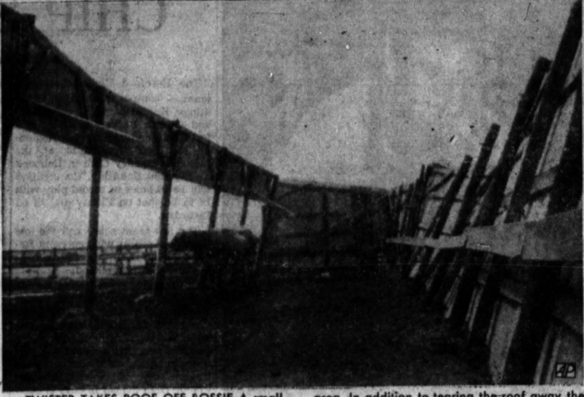
TWISTER TAKES ROOF OFF BOSSIE A small tornado near Houston left this cow without a roof over her head when the top of this large shelter was lifted and scattered over a large area. In addition to tearing the roof away the wind also pushed outward the walls of the structure. (AP Wirephoto).
