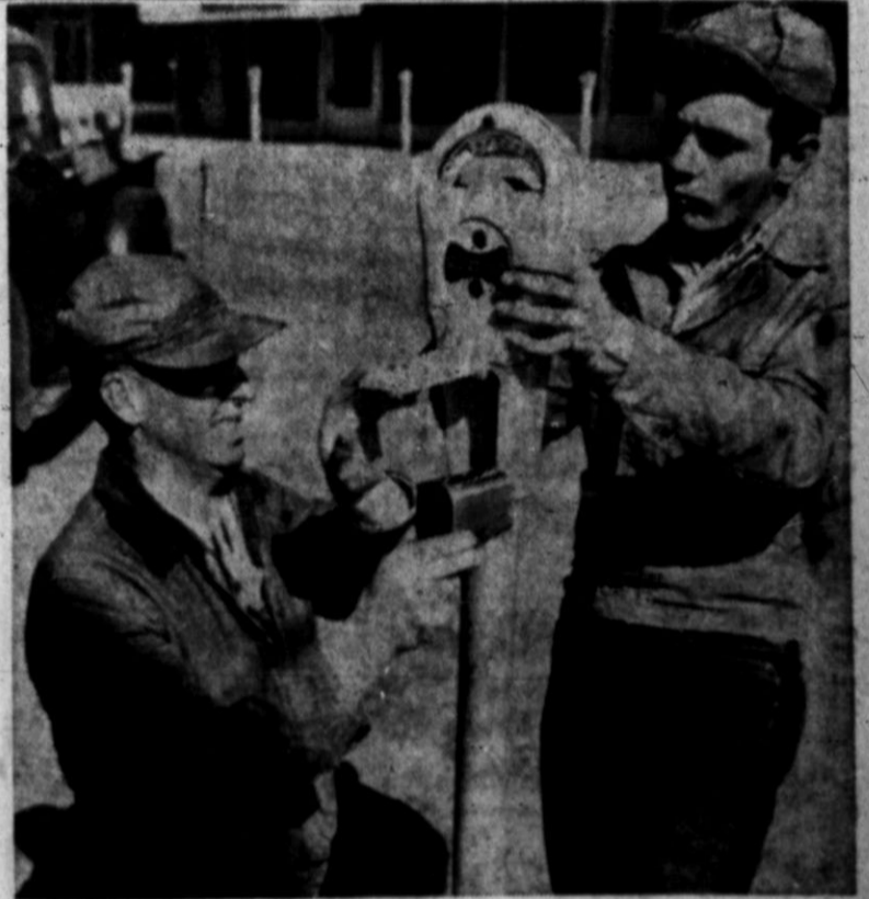
IT'LL WORK NOW! New, late model parking meter heads went on 215 posts in Hereford this week, replacing worn heads which led customers to the universal complaint, "I put in a penny, but the meter wouldn't work." Making the station above are C. M. Leffel (left) and Jack Willier, Staff Photo.
