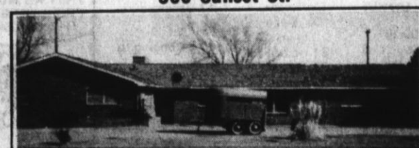
Circle drive and rear entry garage, antique brick, formal living room with 2 fire places, $85,000.00
