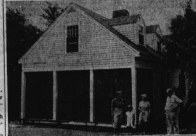
verted into a sixroom house, above. The roof line was extended, and fire-re-sistant asphalt shingles took the place of the worn ammable roofing. Dormers give more light to the upstairs.
