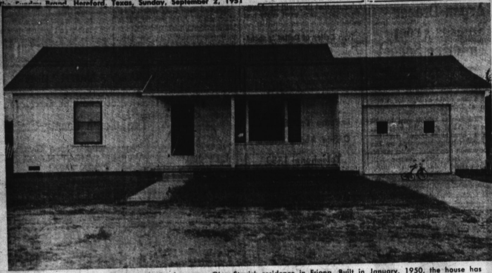
A CARPENTER'S IDEA of a home is the four-room Glen Stevick residence in Friona. Built in January, 1950, the house has extra large bedrooms and sliding doors throughout. The Stevick laundry is in the garage. This is the second home the Stevicks have built. Their next one will incorporate the newest home building kinks.—Brand Staff Photo.
