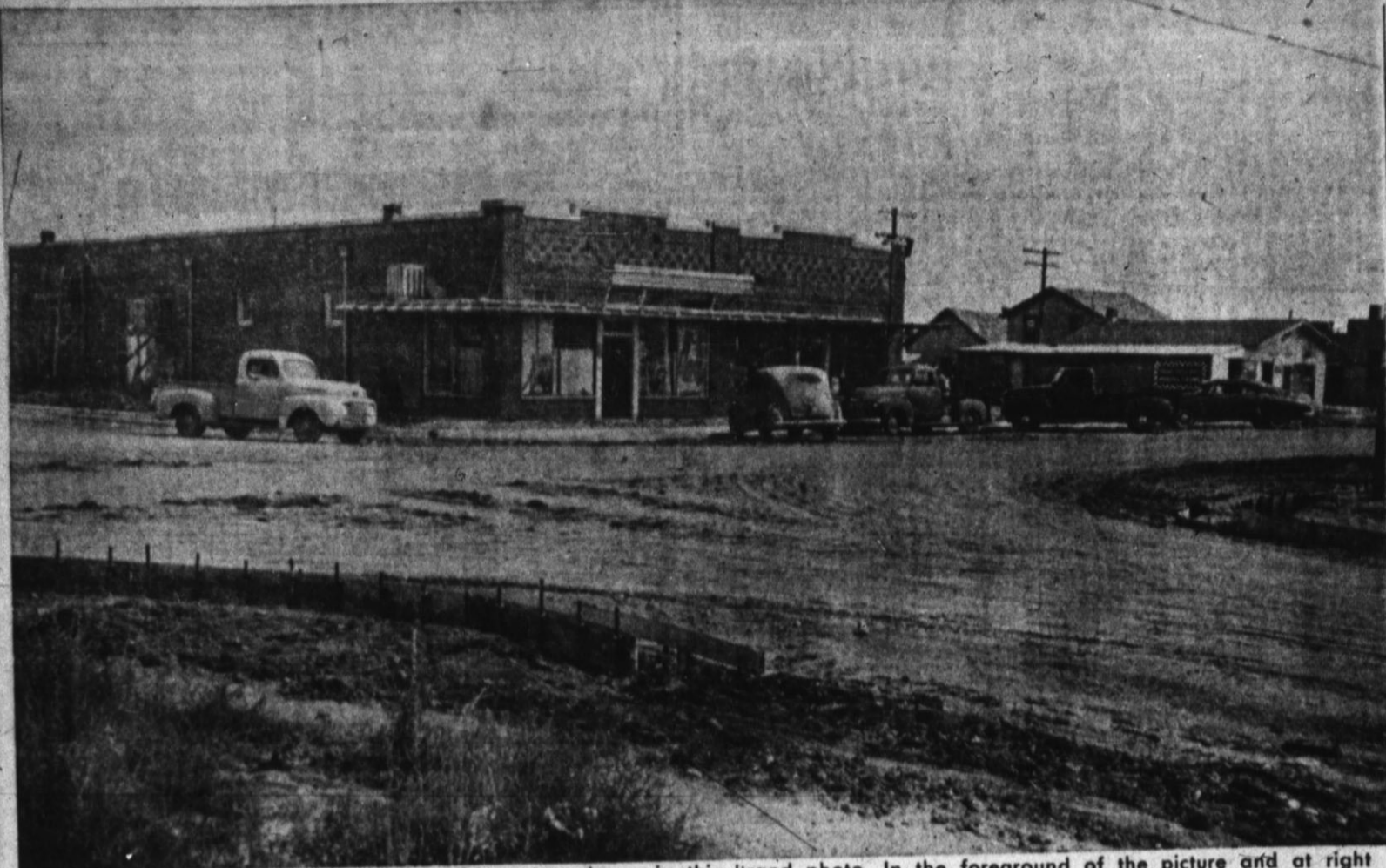
THE OLD AND THE NEW views at Friona are shown in this Brand photo. In the foreground of the picture and at right can be seen paving gutter forms for laying the new pavement in Friona. In the background is a completed curb and gutter around the corner.—Brand Staff Photo.
