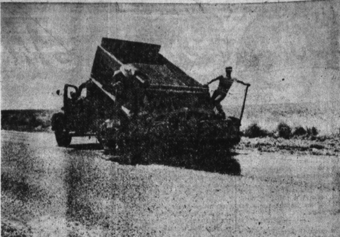
WORKMEN FOR Bell, Braden, Barker and Gilven, Amarillo contractors are shown putting the rock topping on the new Farm-To-Market road running nine miles north of Smith. Cpl. Wolfe is stationed at Fort Sill, Okla. Airman and Mrs. Junior Murrell of Amarillo spent the week-end with Mr. and Mrs. Virgil Lamb.
