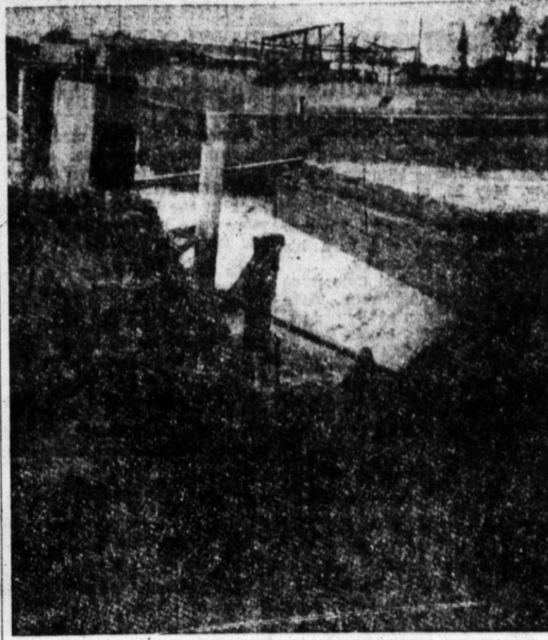
HEAVY RAINS washed out this concrete-slab bridge on New York street this week. Leland Alderson Photo.
