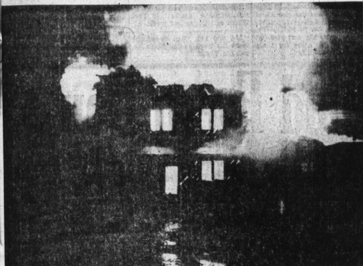
FRASER'S FEED MILL suffered the same fate as the flour mill—only about 15 minutes later. This picture shows the mill as flames leap high as the structure was undergoing complete destruction. Brand and Bill Patton Photo.
