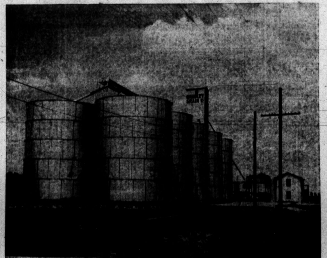
BRADLEY GRAIN ELEVATOR
