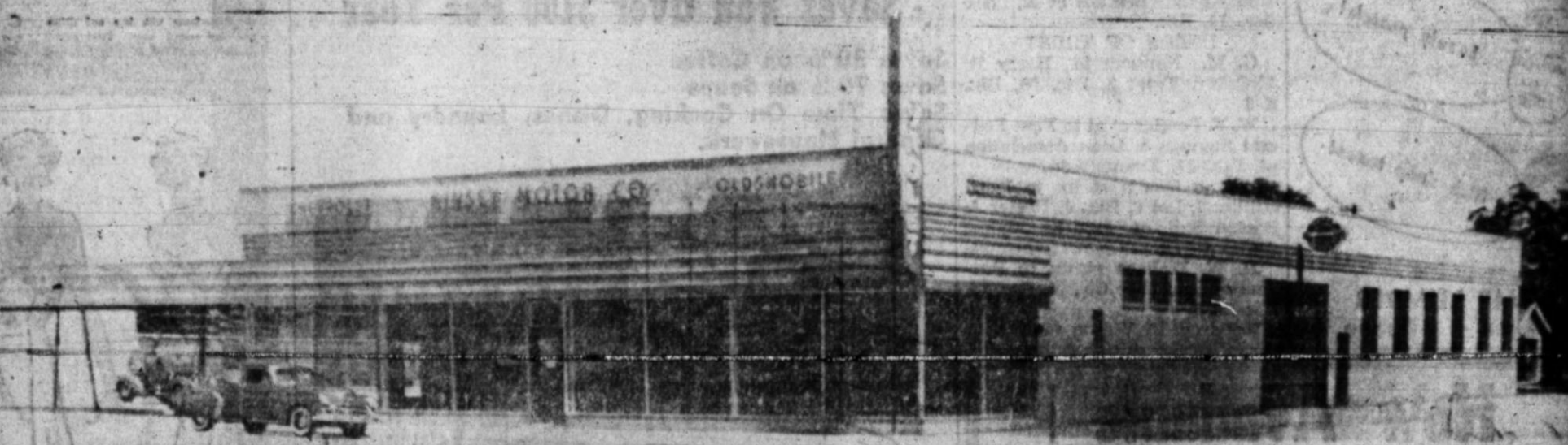
EXTERIOR VIEW NEW KINSEY MOTOR BUILDING
