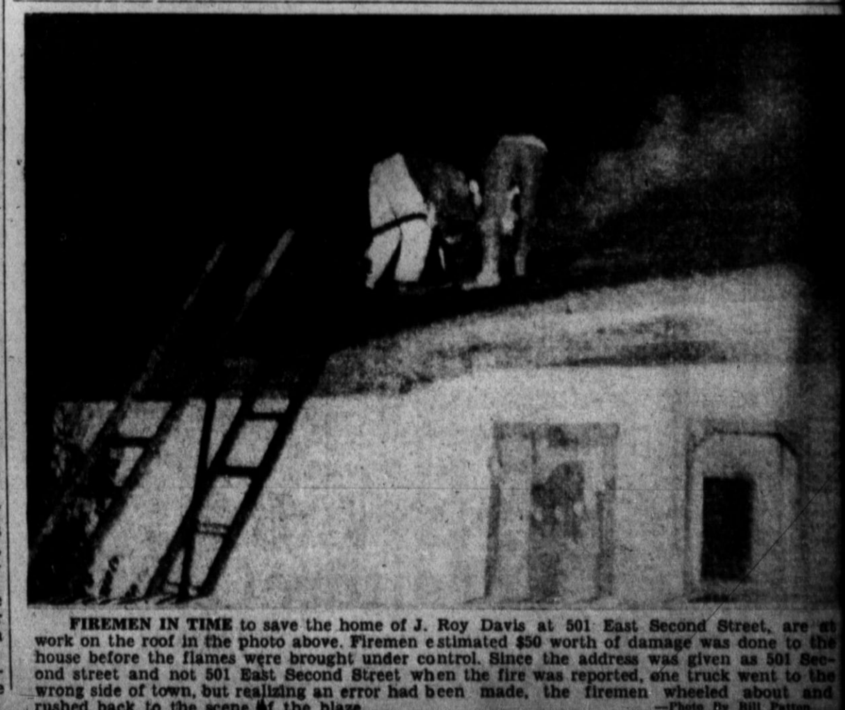
FIREMEN IN TIME to save the home of J. Roy Davis at 501 East Second Street, are at work on the roof in the photo above. Firemen estimated $50 worth of damage was done to the house before the flames were brought under control. Since the address was given as 501 Second street and not 501 East Second Street when the fire was reported, one truck went to the wrong side of town, but realizing an error had been made, the firemen wheeled about and rushed back to the scene of the blaze. —Photo by Bill Patton
