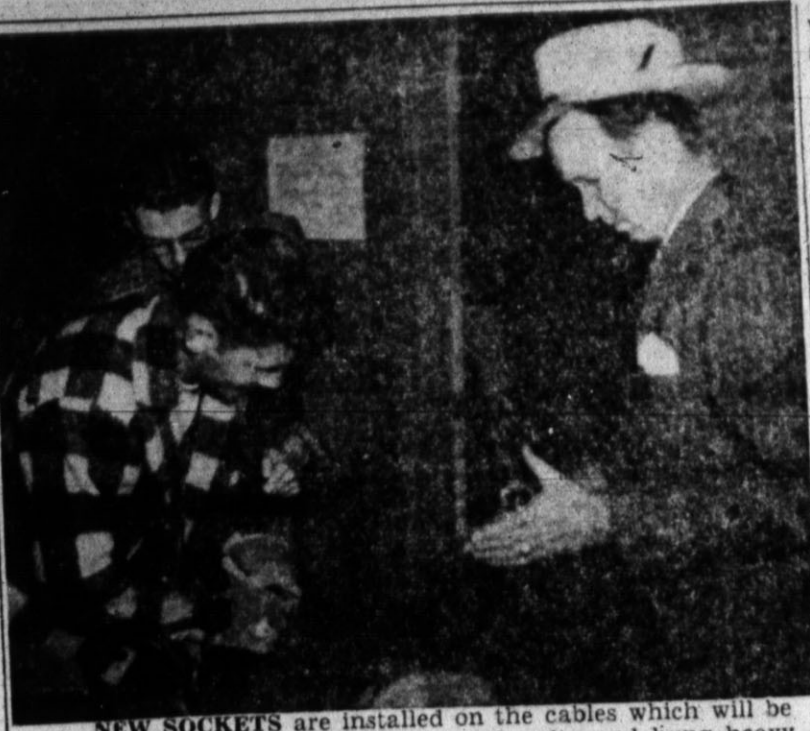
NEW SOCKETS are installed on the cables which will be strung up and down the streets of the city and hung heavy with brilliant lights to give the town a Yuletide atmosphere. Left to right, Otis Hall, Bill Howard and Nolan Grady. —Brand Staff Photo
