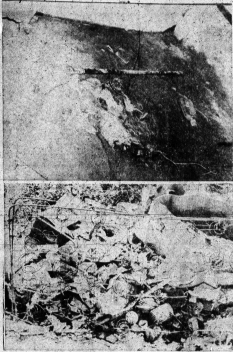
HERL'S WHY County Health Officer Dr. L. B. Barnett found the men's shower at the Hereford Labor camp looking like the top picture and "bed spring" trash containers that cannot be emptied any way except by hand in his inspection of the Camp Wednesday before he made several recommendations to help the fly and health situation in the Hereford area.
