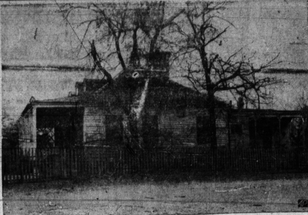
FRENCH LEGATION BUILDING —This was the French Legation Building in Austin during the days of the Republic of Texas. It is a crumbling relic of the era when the French Minister to Texas was his Excellency the Right Honorable Count Mons. A. Saligny. Maury Maverick of San Antonio is campaigning to get the City of Austin and State of Texas to restore the old French Legation building before it's too late. (AP Photo)
