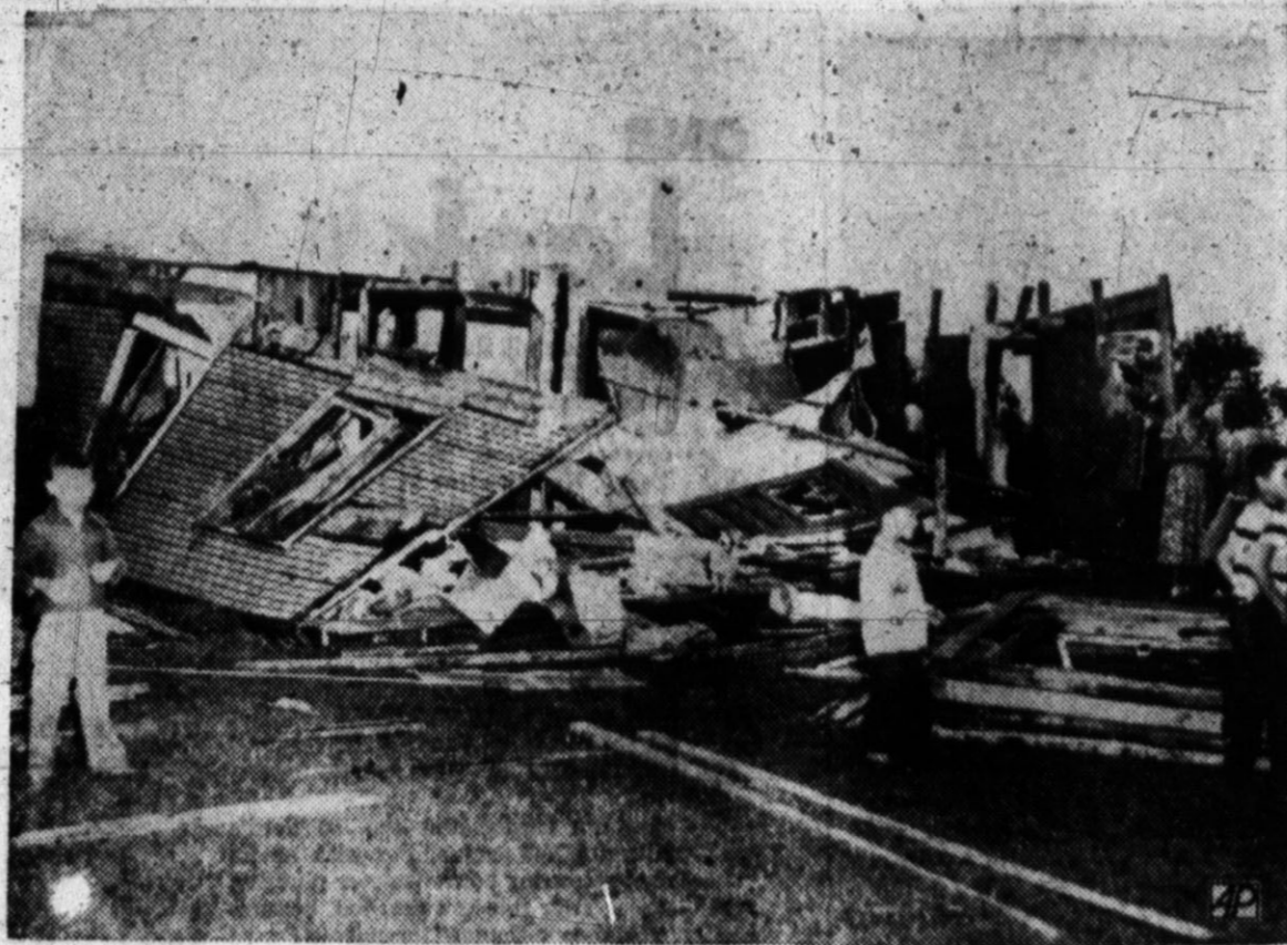
STORM WRECKS HOME —The home of O. L. Fagan lies in ruins near Denton after the passage of gale-like winds on May 29. Property damage was heavy over a large section of the state after storms ripped through. (AP Photo)
