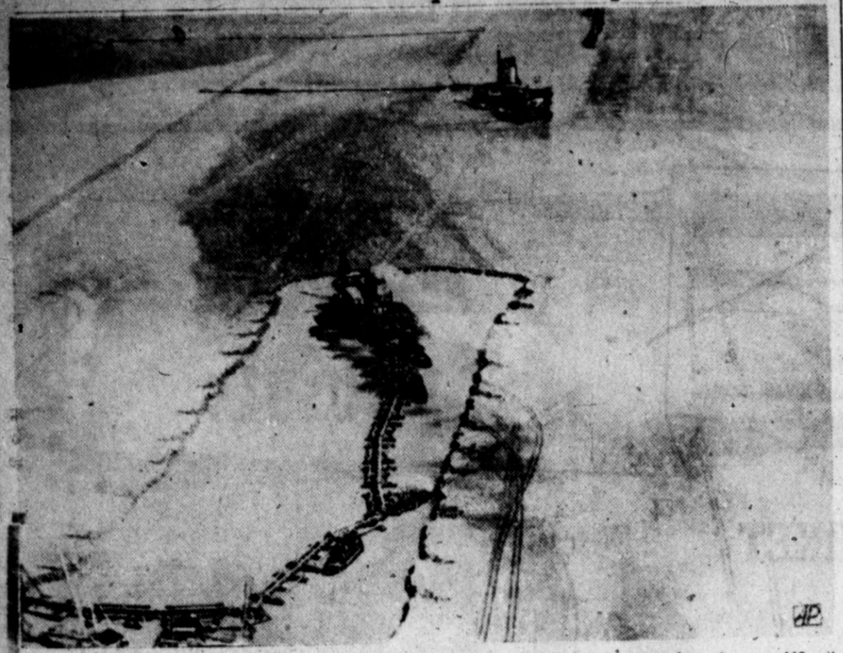
The dredges Miami and Caribbean are some 900 feet apart as they bring to an end work on a 112-mile section of the Gulf Intracoastal Waterway that has been under construction since January, 1946. They met about 7 miles south of Corpus Christi, Tex. Ceremonies marking the opening of the waterway connecting Corpus Christi and Brownsville, Tex., were held May 18. The intercoastal system links the Great Lakes area with the Mexican border. (AP Photo)
