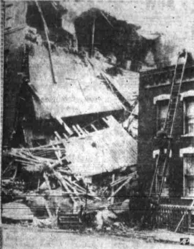
FACTORY WALL COLLAPSES —A brick factory's rear section which collapsed in Chicago buries an automobile among the debris. Firemen at right scale a ladder up an adjoining building to investigate the huge pile of debris. The building is occupied by the Goodman Yarn company and is located on the near southwest side of the city. Six persons were reported injured in the collapse. (AP Wirephoto).
