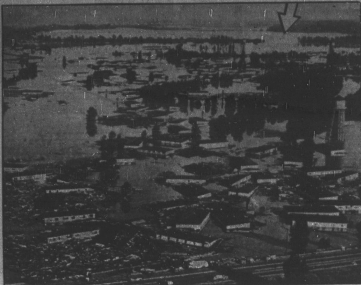
This aerial view of Vanport City, Ore., shows the devastating wreckage of the nation's largest housing project, with debris and whole six-unit, two-story apartments floating in the murky floodwaters of the Columbia River. Arrow points to the breakthrough in the dike wall that surrounds the city.
