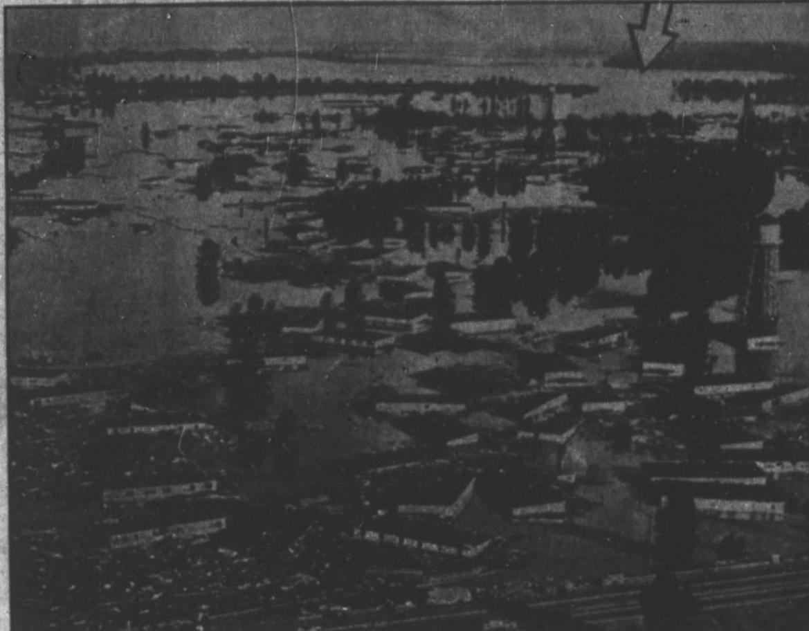
This aerial view of Vanport City, Ore., shows the devastating wreckage of the nation's largest housing project, with debris and whole six-unit, two-story apartments floating in the murky floodwaters of the Columbia River. Arrow points to the breakthrough in the dike wall that surrounds the city. Damage was estimated at $27,000,000.
