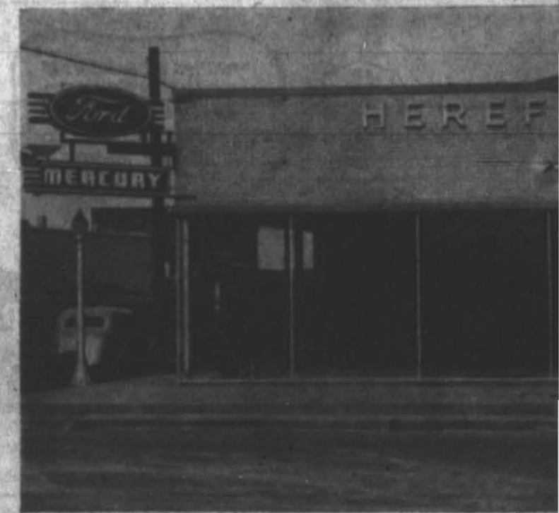
This Miles Street front of the Hereford Motor Company embraces making the entire show room, offices, etc.
