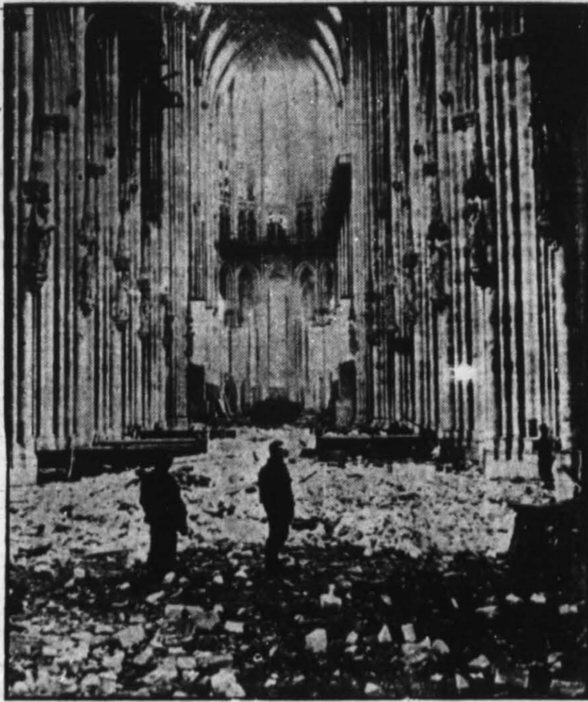
American soldiers survey damage in famed Cologne Cathedral—a litter of masonry from upper regions of the edifice. The Gothic pillars appear undamaged.
